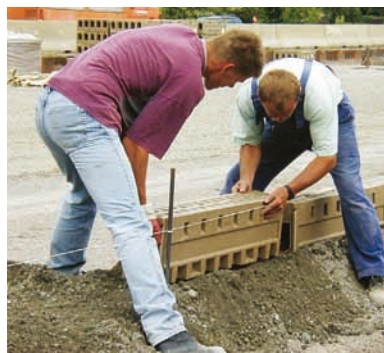
ACO DRAIN® Monoblock RD 100 – easy to install without lifting gear.
