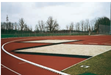
ACO SPORT system 7000 Sand trap channels and elastic perimeter kerbs enclosing the long jump pit. They hold back the sand and keep the running track clean.
