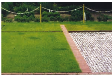
Parking space reinforced with grass grid
