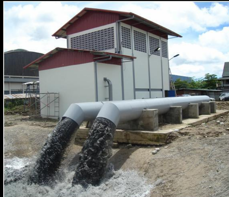
23 Vertical Turbine Pump Sets Across 9 Pumping Stations For Irrigation & Dewatering
